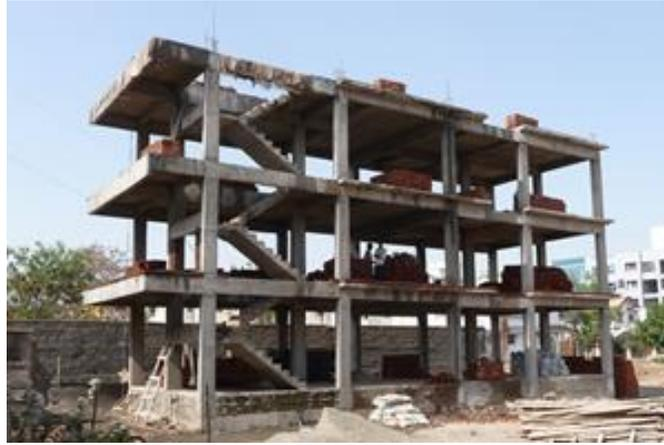
*Figure 2. The reinforced concrete floors of this building tie the beams and columns together and force all these parts to move together horizontally during an earthquake.*
